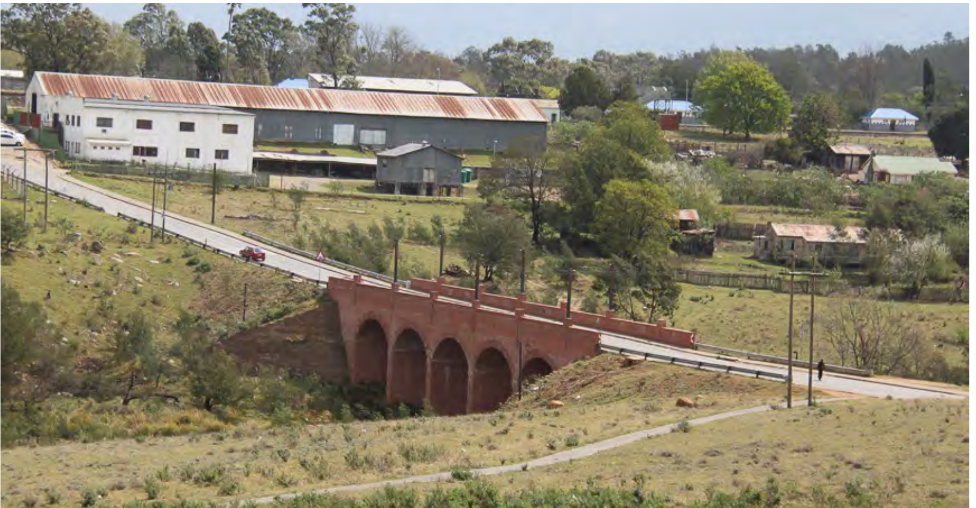
BRIDGE BUILDING: The NCOP delegation inspect the Kraaipan bridge, which was damaged during heavy rain in January this year.
