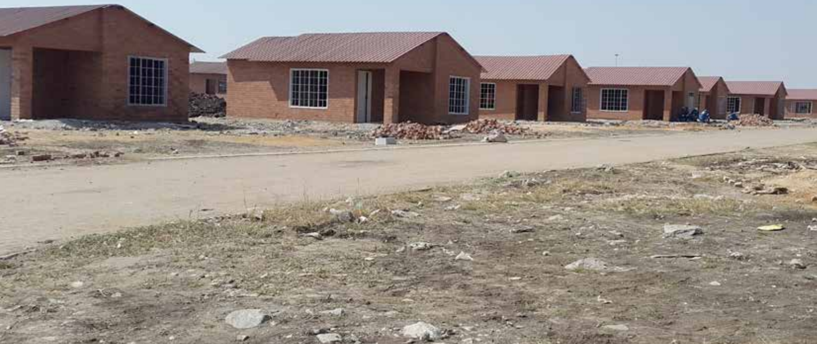
BREAKING NEW GROUND: The completed phase 1 of the housing project in Marikana Extension 2 in North West.
