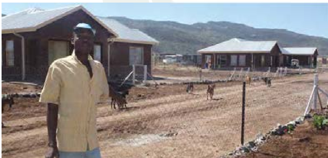
SUCCESS STORY: Some of the 42 houses that were built in Monametse, Limpopo, following concerns raised by the community during the TPTIP programme held in 2010.
