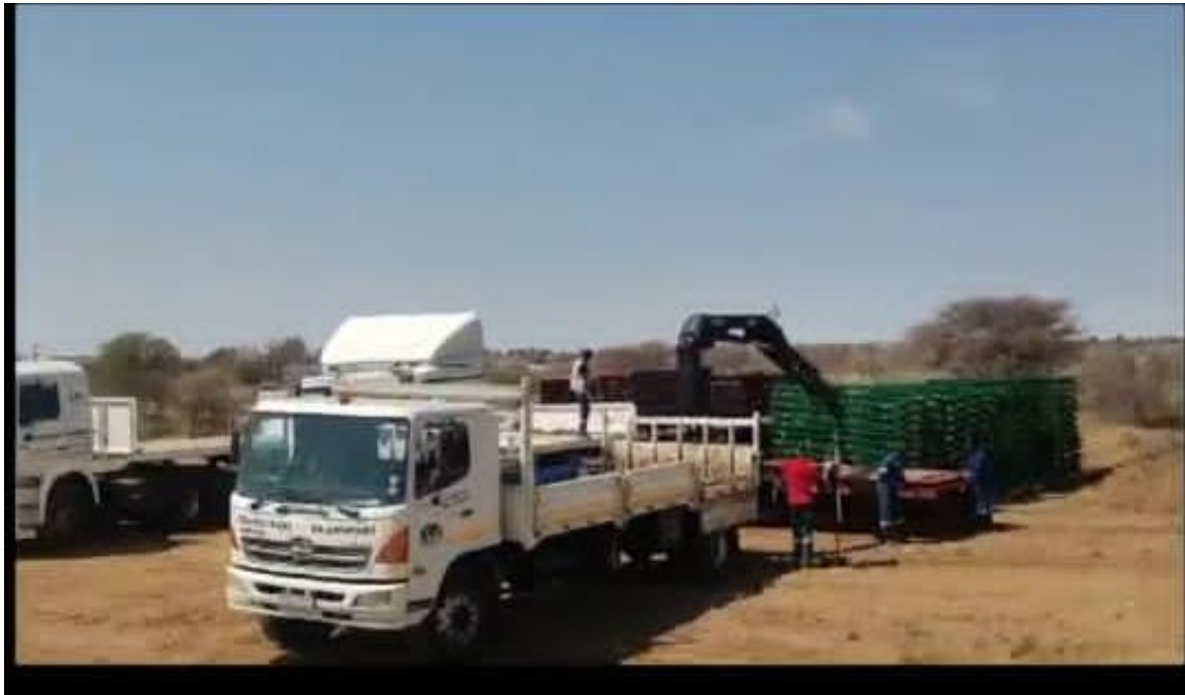
Offloading of bridge components
