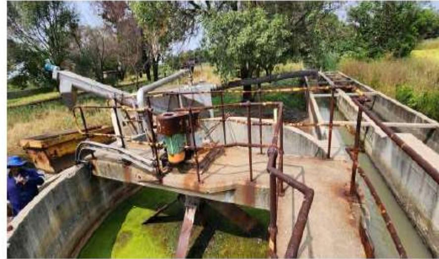
After: New Grit Continuous Flow Receiver and pipe work installed. (Functional)
