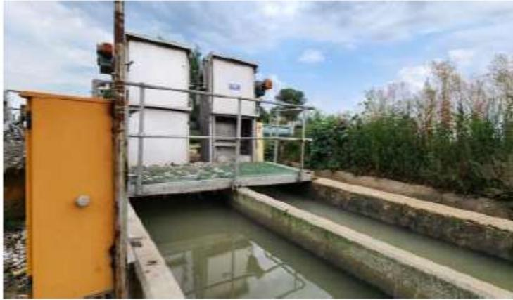
After: New Coarse Mechanical Front Rakes. (Functional)
