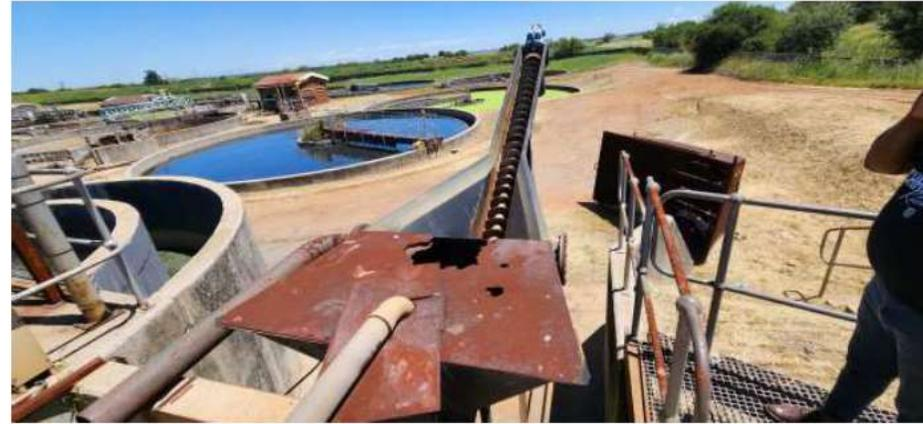
After: Grit Classifiers completed with discharge pipework. (Functional Grit Classifier)
