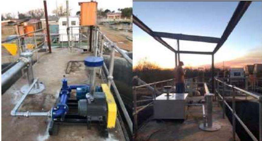
Before: Grit Classifiers complete with discharge pipework. (Non-functional Screen)
