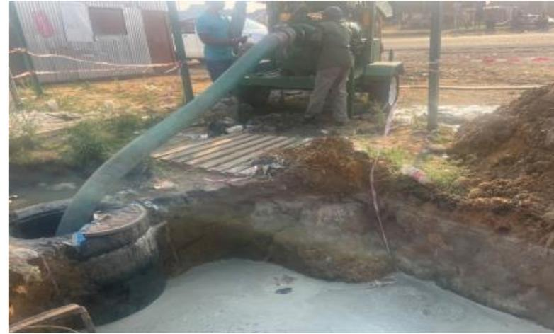
Pumping sewer waste out in preparation for fixing collapsed sewer in Kutlwanong
