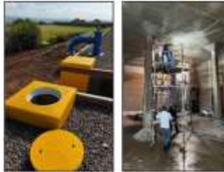
LEFT: Refurbished KwaMakhutha tanks.
