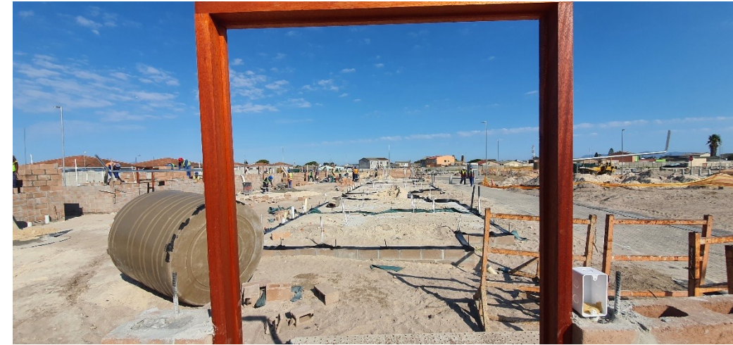
Figure 4: Completion of services and start of top structure construction.
