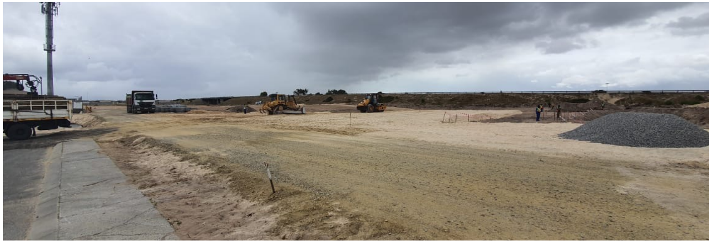
Figure 3: Farm 694 Earthworks – October 2019.
