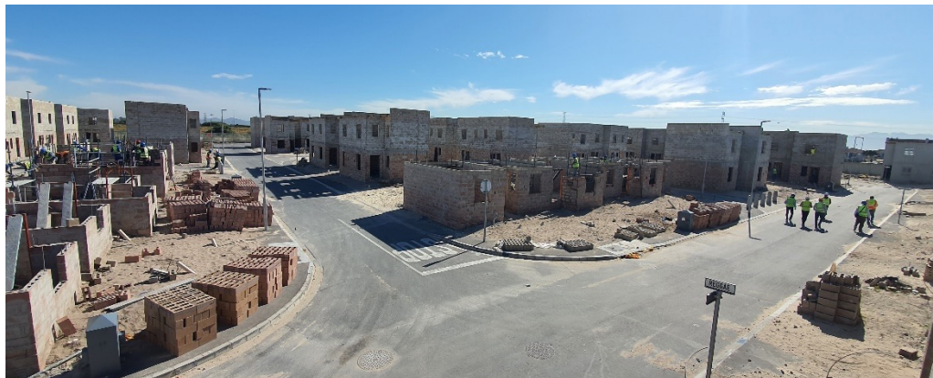
Figure 5: Top Structure construction - September 2021.
