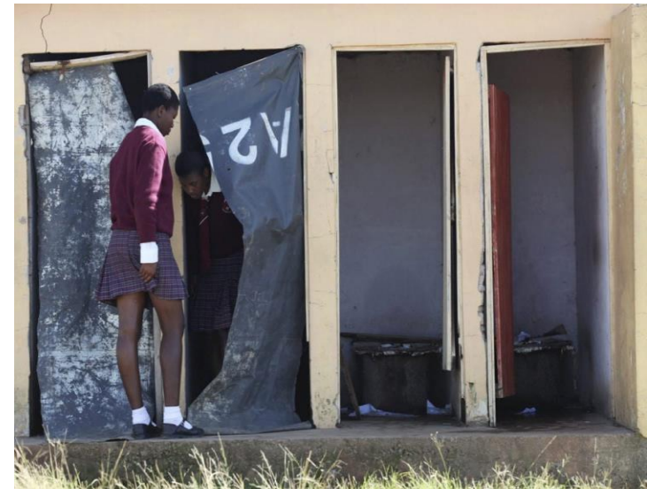
Pit latrines at an E. Cape school
