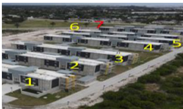
Nelson Mandela University – bird's eye view of student accommodation (blocks 1 to 6 completed for occupation in February 2023)
