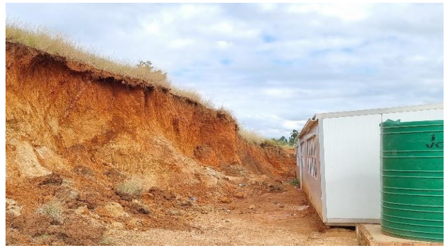
Placement close to steep embankment
