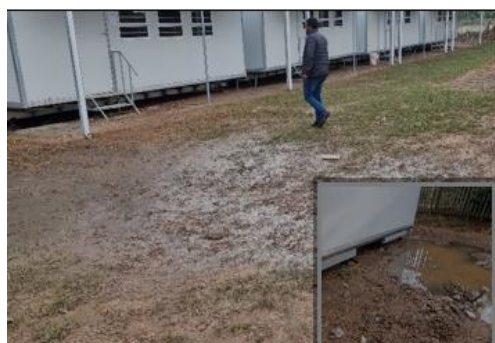
Mobile units constructed on land previously submerged by floods
