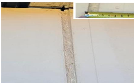
Gap (2,5 cm) between wall panels filled with sealant
