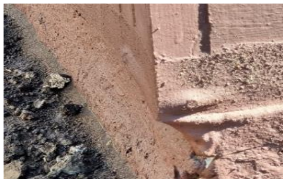
Wall panels positioned outside concrete slab's edge
