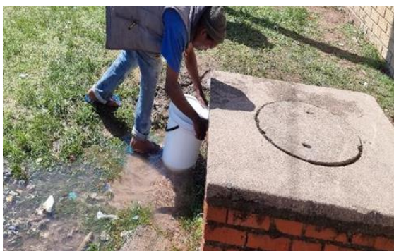
Overflowing manhole used as source of water in KwaDabeka
